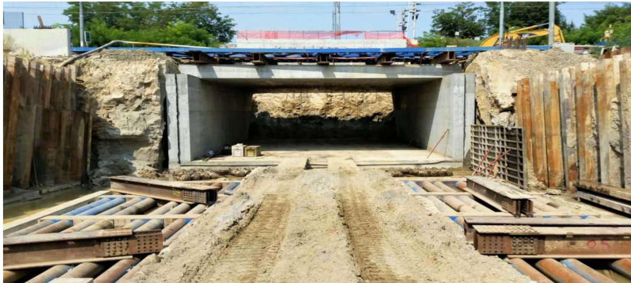
Taking water pipeline through railway underpass
