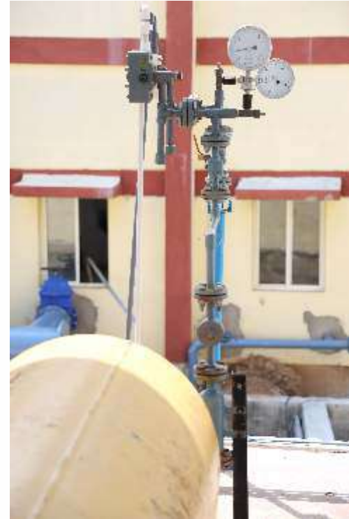
Chlorination System at Water Treatment Plant in Banda
