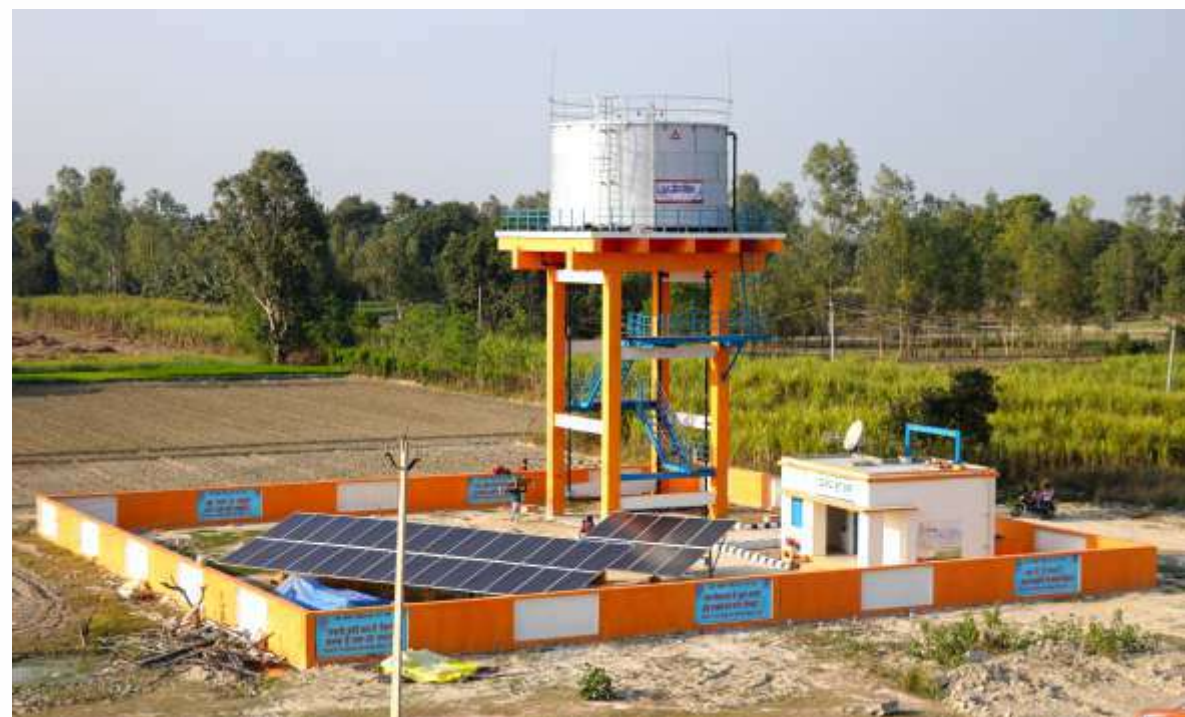
Overhead Tank in Sultanpur powered by Solar Panels
