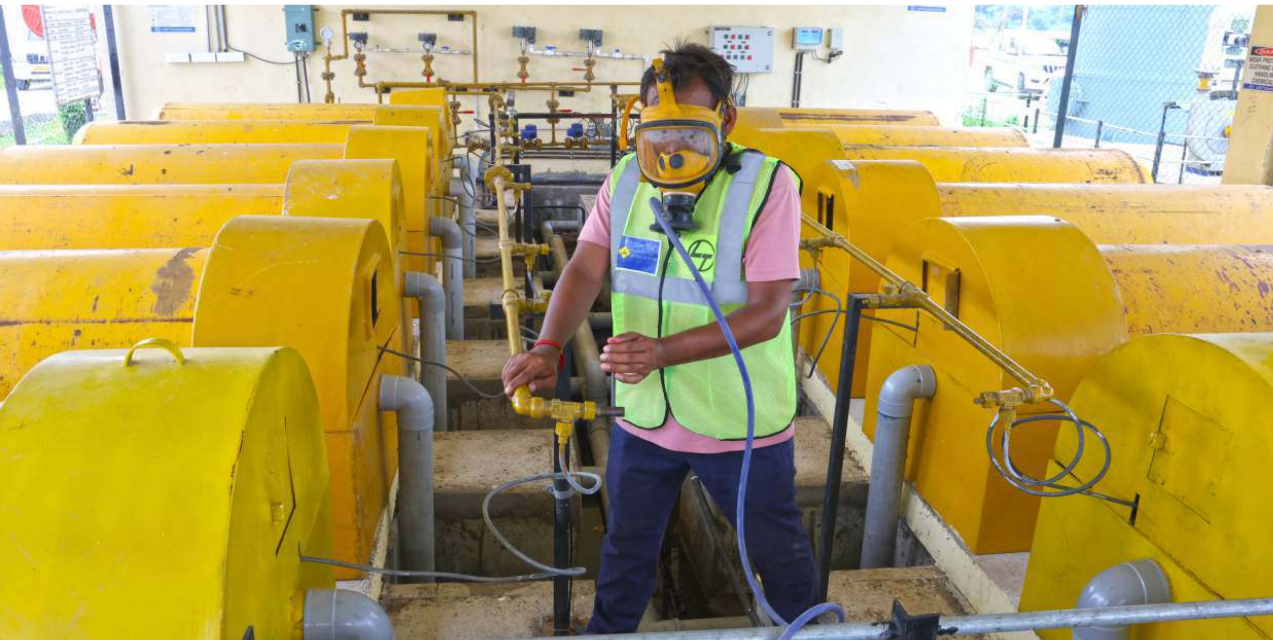
Chlorination System at Water Treatment Plant in Banda
