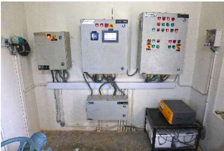
Chlorination and Automated System at OHT, Ghazipur
